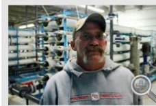
Creighton, Nebraska water operator, Kevin Sornhisen, stands before the $1.3 million water filtering system.
