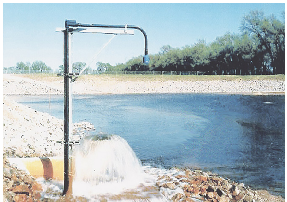
Figure 6. Recharge basin where water from the Little Arkansas River is recharging the Equus Beds portion of the High Plains aquifer.
