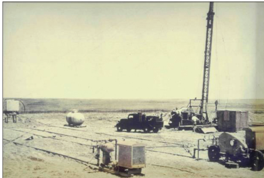
Figure 1—First experimental fracturing job conducted in 1947 by Stanolind Oil in the Hugoton gas field of southwestern Kansas utilizing “1,000 gallons of naphthenic-acid and palm-oil- (napalm-) thickened gasoline” . . . “and sand from the Arkansas River” (from Montgomery and Smith, 2010, p. 2).
